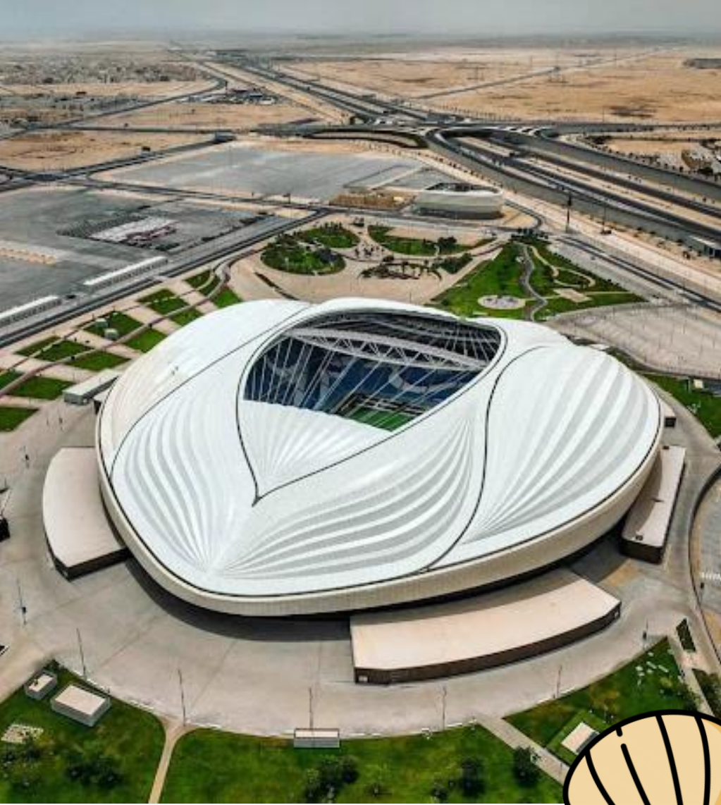
Al Janoub Stadium
